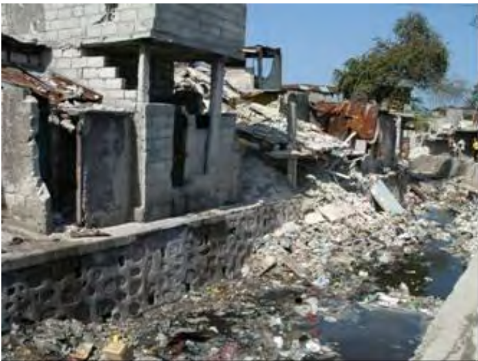
Debris and waste filling water canal in downtown PAP – disease vectors increase.
