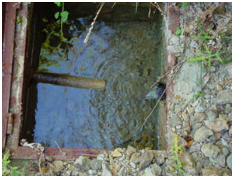
Photograph 5.4: Part of Haret-Jandal spring diverted into potable water network.
