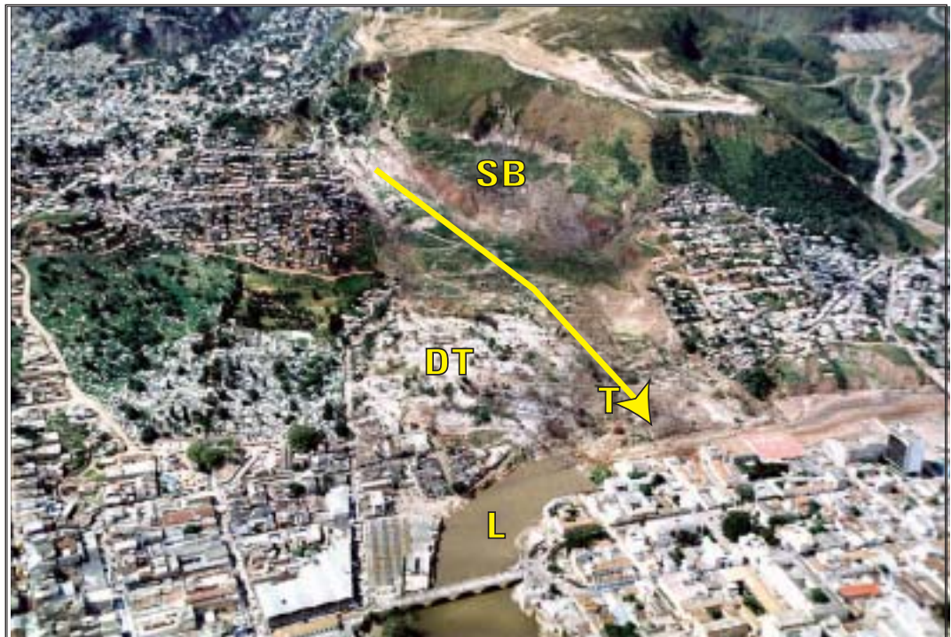
Figure 2. Aerial view of the El Berrinche landslide, a complex slump/earth flow that dammed the Río Choluteca in Tegucigalpa. The arrow indicates the direction of movement of the earth-flow tongue. "T" denotes the toe of the landslide that dammed the river, and "L" indicates the lagoon dammed by the toe of the landslide. "DT" indicates the highly deformed toe of the landslide where the center of Colonia Soto was, and "SB" denotes the upper slump block.
