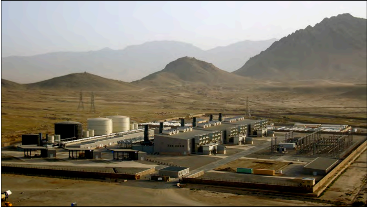
The Tarakhil Power Plant, located on the outskirts of Kabul, has 18 diesel generators capable of generating 105 megawatts of electricity. (Photo from mission archives, September 2010)
