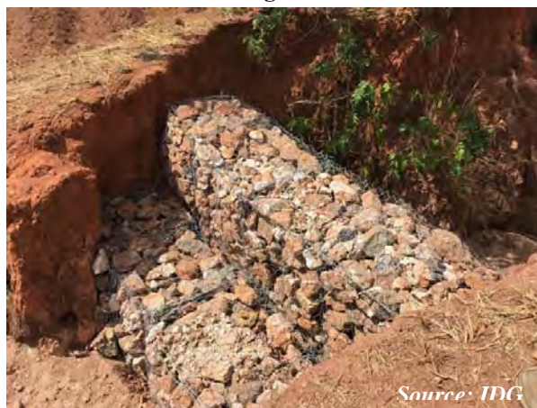
Figure 27: Gabion constructed in the Dedza region
