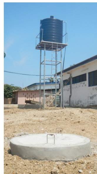
The underground geodesic dome (foreground) and above ground water storage (background) provided to the State School for the Deaf at Adjei Kojo.
