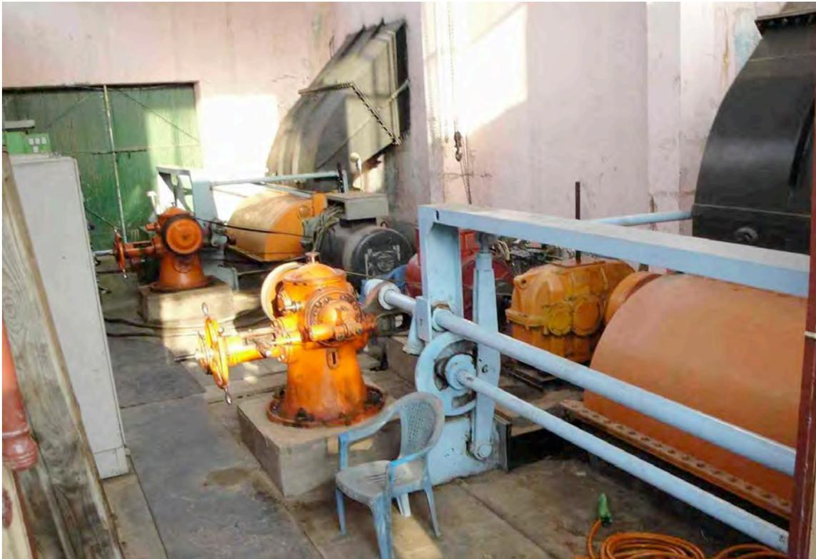
**Fig. 4. Asad-Abad powerhouse with 2 crossflow turbines producing ~185 kW each.**
