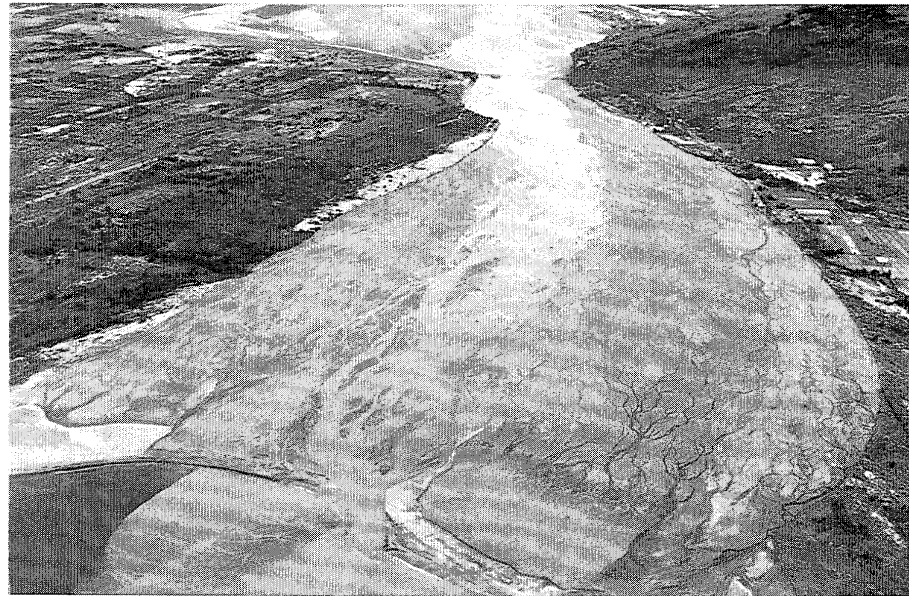
Sediment deposition at the river's mouth, Highway 7 bridge in background, February 1993.
