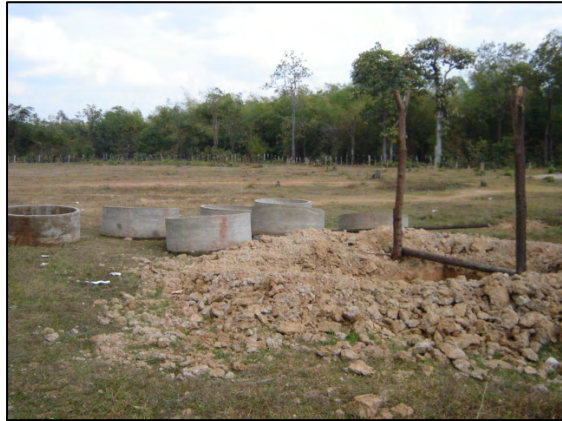
Building a ring well at a village school
