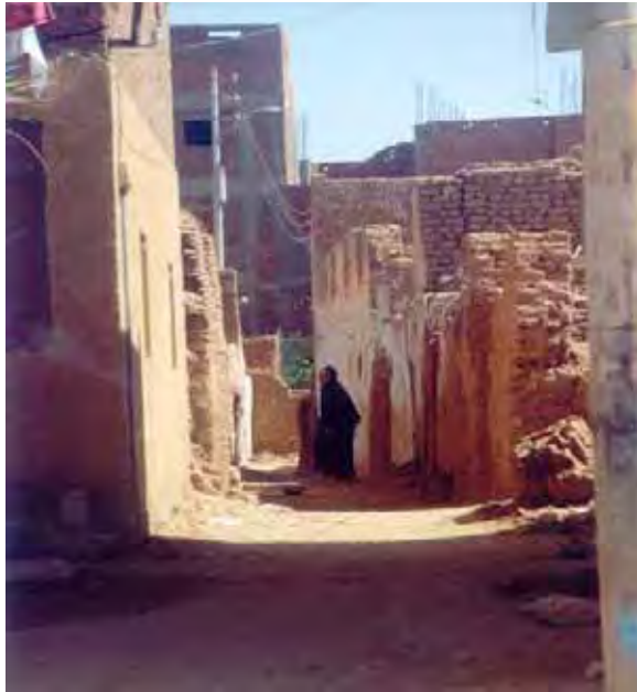
Figure 17. Typical El Gedida Street
