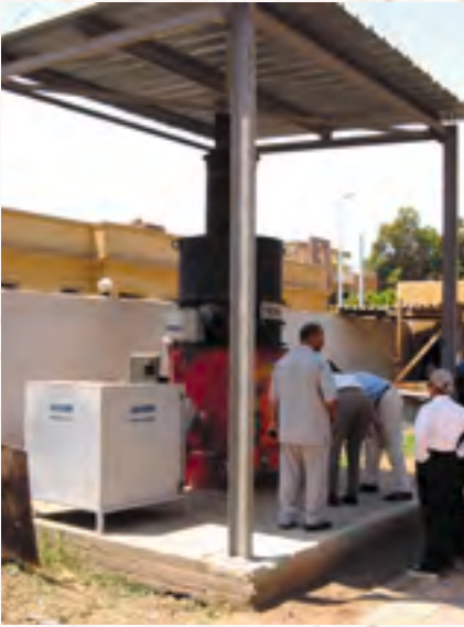
Medical waste facility in Luxor.
