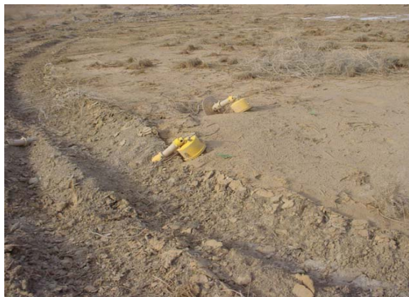
Damaged Approach Lights RWY 33R
