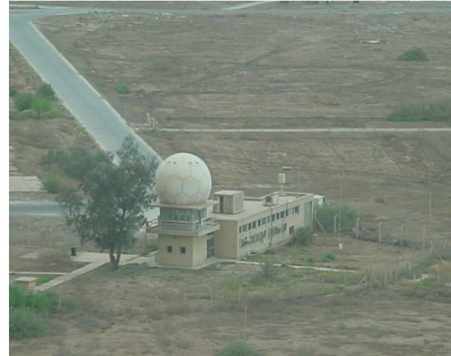
Weather Station – View from Control Tower
