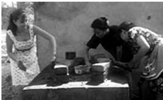
Community women building a Finlandia stove
