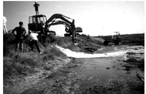
Managed retreat in progress in the Blackwater Estuary, Essex, UK. Tidal water is entering a grazing marsh for the first time since its reclamation in 1750
