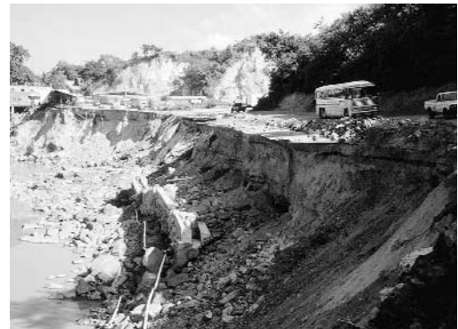
Landslide in Honduras
