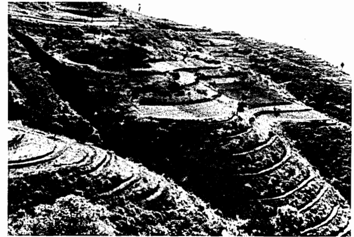
Figure 4. Results of the extensive soil conservation campaign in Ethiopia funded by the World Food Programme. Small terraces were constructed for reforestation and contour bunds for plowed land that should develop into graded terraces in the course of decades. M. Coendet, Harerge region, March 1982.
