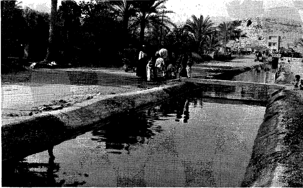
PHOTO 1. BENI MAGDUL CANAL LINING
