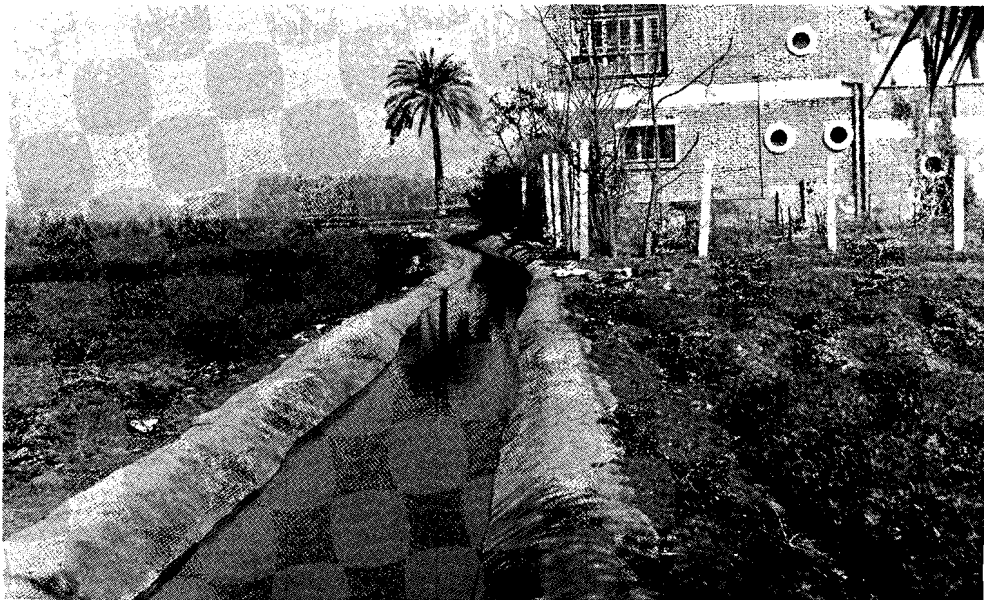
PHOTO 5- LINING WITH RUBBER SHEETS PRODUCED BY TAURUS RUBBER WORKS COMPANY
