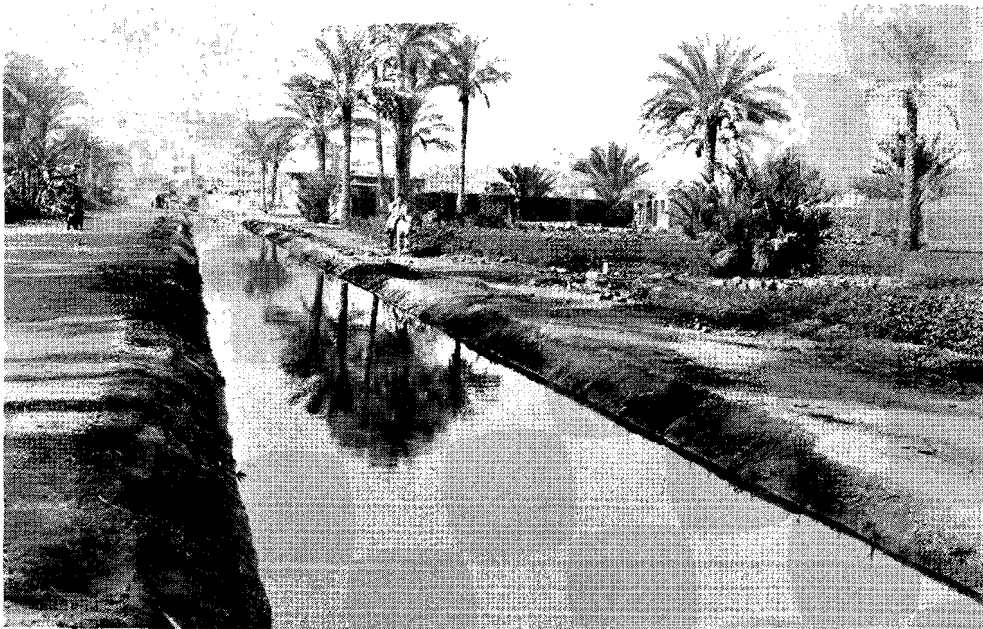
PHOTO 2 - BENI MAGDUL CANAL LINING
