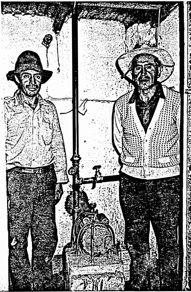
Inside pump house.
