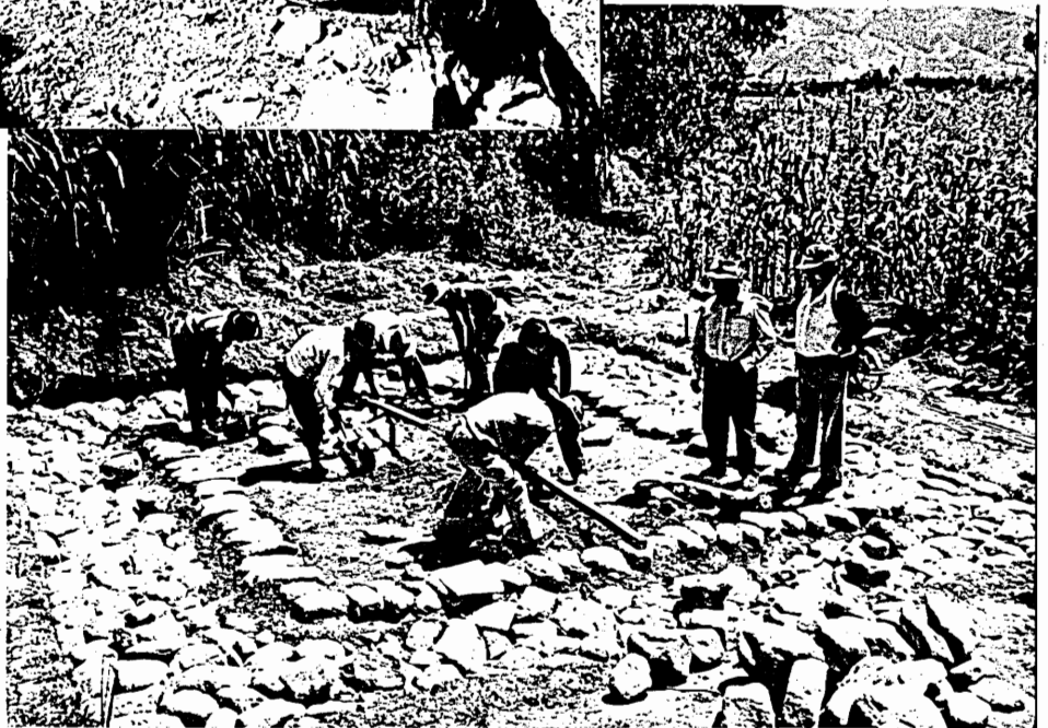
Masonry storage tank under construction.
