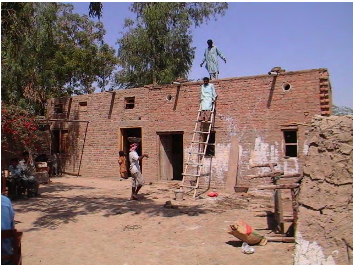
Communities and local masons working together to improve a school's infrastructure.
