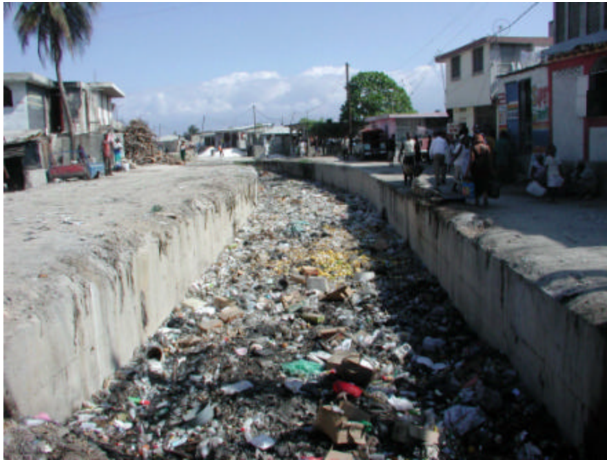
Drainage Canal – Downtown
