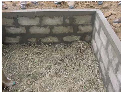
Curing chamber floor covered with straw
