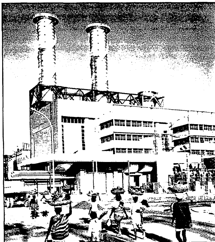
Donaldson inlet filter system on NTPC Gandhar gas turbine power plant in Gujarat.
