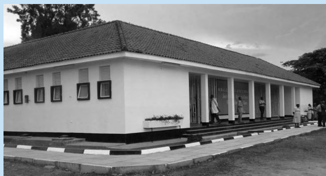
The Mbale Hospital JCRC AIDS Clinic underwent renovations with support from the Emergency Plan, providing the clinic with the capacity to conduct sophisticated tests required in ART management and monitoring that were not previously available.
