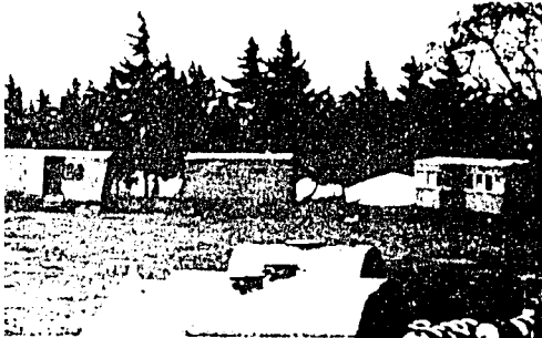
Highway Caravan on wheels at Çardak near Dardanelles. Caravan is fitted out to construct highway stretch without outside assistance.
