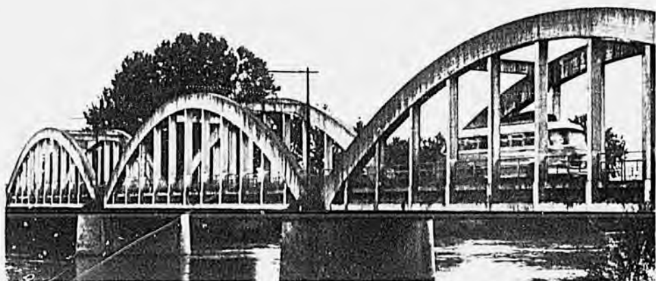
Sakarya River highway bridge.
