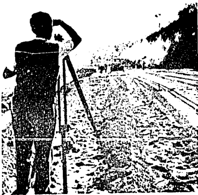
Engineer at work on the new Ordu-Giresun-Trabzon highway.
