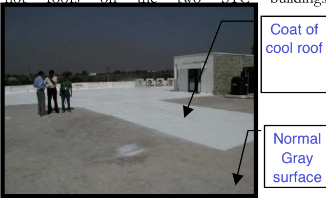
Figure 1. Installation of cool coating on the concrete roof, and kWh consumption with respect to outdoor and indoor temperature difference
