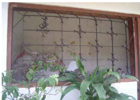
Figure 8 Storage room of recyclables
