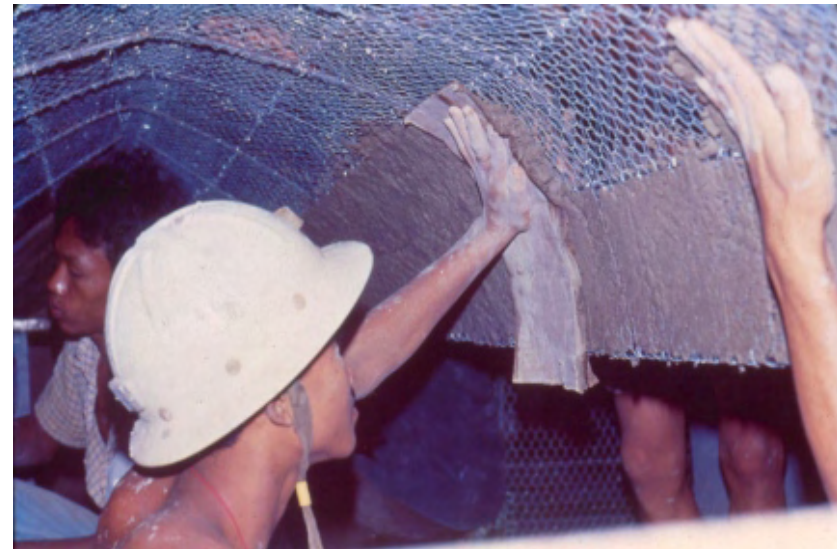
Fig. 5.4 Ferrocement construction process (photo: IFIC)
