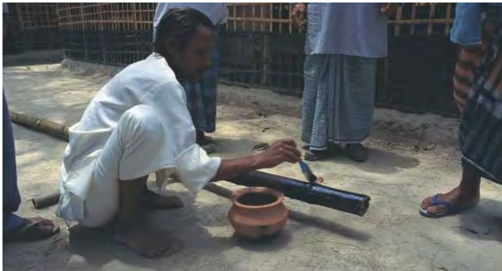
Fig. 2.4 Painting lower end of bamboo post with bitumen
