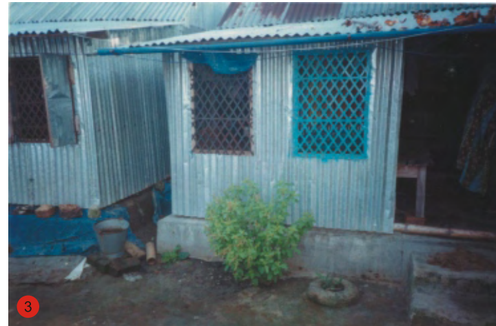
Fig. 2.1 Cement-stabilized earthen plinth
