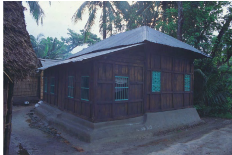
Fig. 5.10 House made of timber in Bhola, where supply of bamboo is limited
