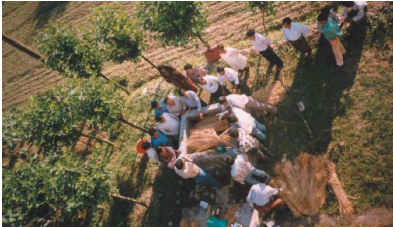
Fig. 2.11 Treatment of thatching material by soaking in chemical preservatives
