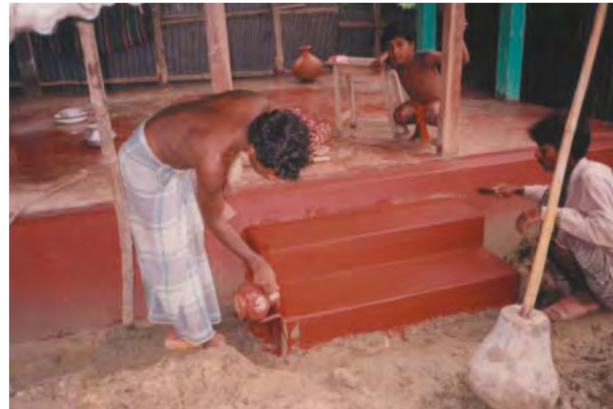
Fig. 2.2 “Dowa-posta” plinth construction
