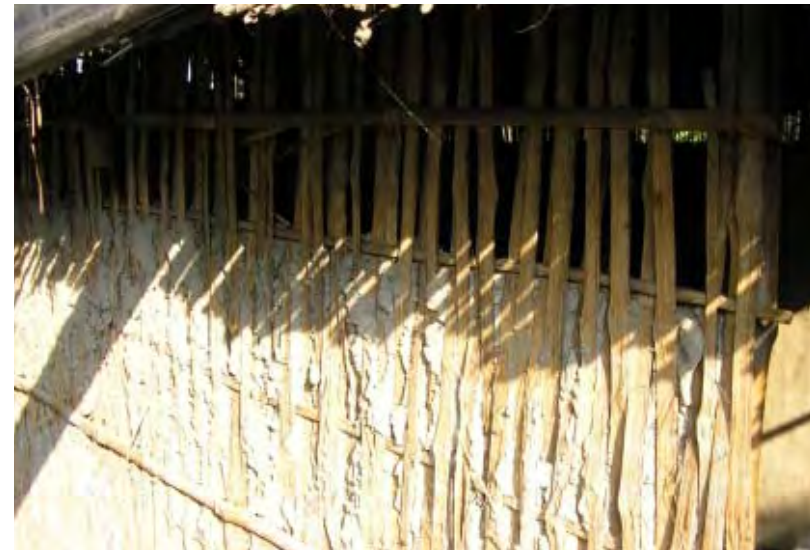
Fig. 4.2 Wall built in the wattle-and-daub method
