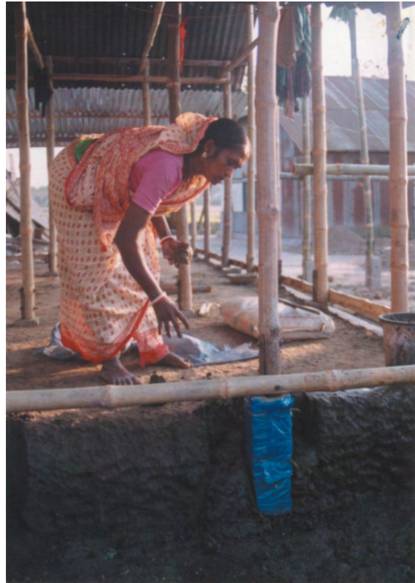
Fig. 2.5 Concrete stump (kaatla) for protecting lower end of bamboo post
