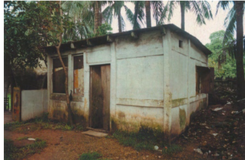
Fig. 5.3 House made of ferrocement wall and roofing panels
