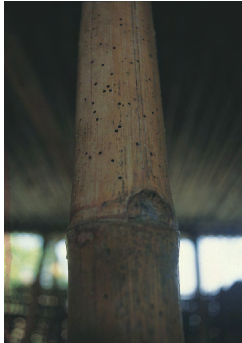
Fig. 3.1 Bamboo post under insect attack
