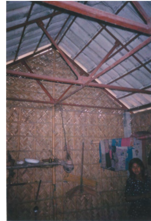
Fig. 5.8 MS angle roof truss used by Caritas (adapted from Caritas) and house with MS angle truss built by Proshika
