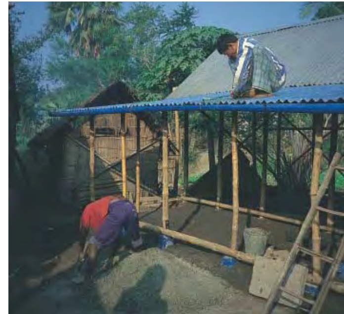
Fig. 2.13 PVC pipe rainwater gutter detail and house being built with a gutter
