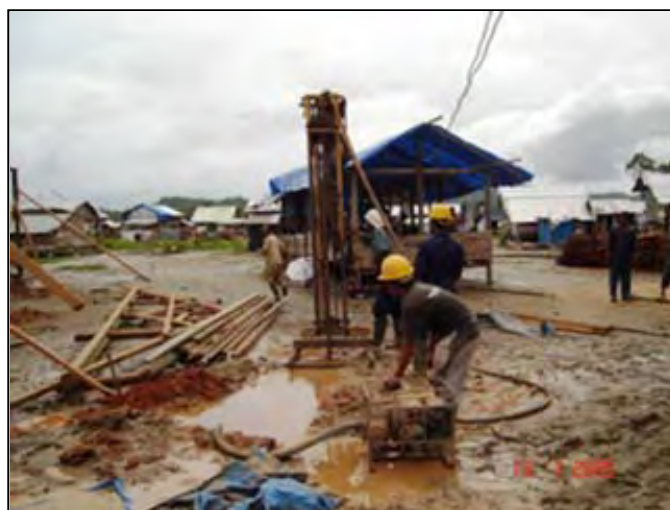
Figure 5: Well Drilling in Aceh.
