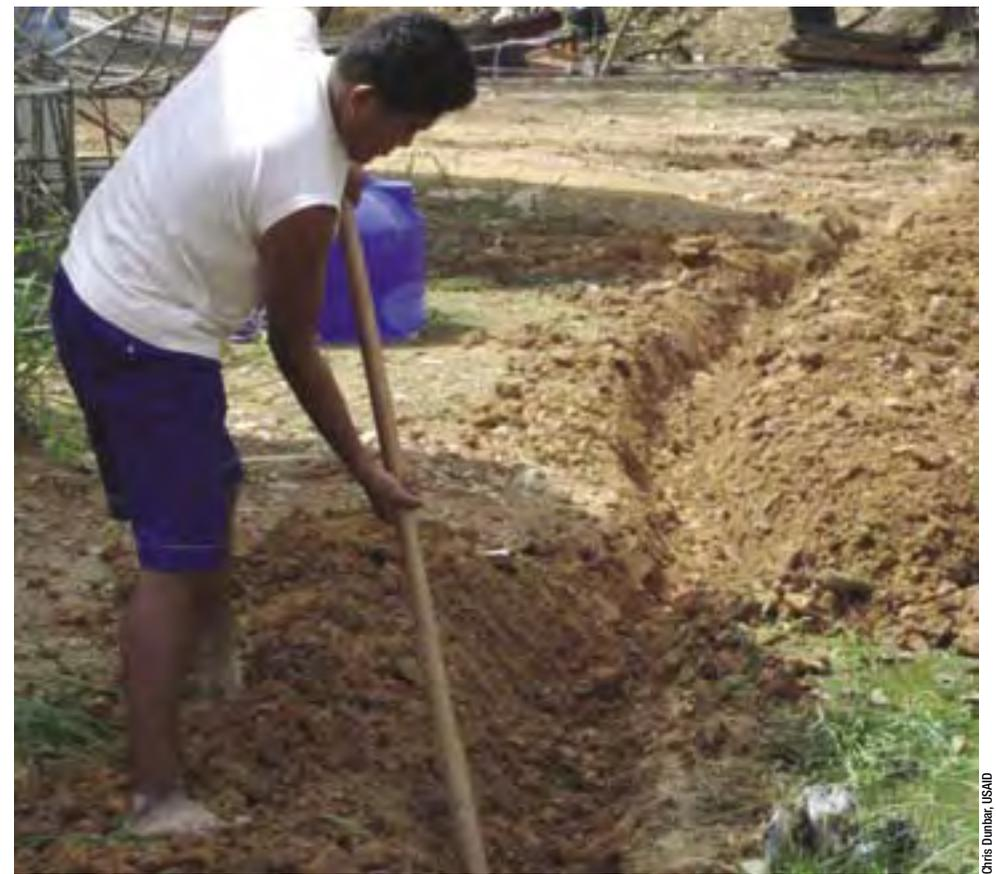
*A villager digs trenches for pipelines to connect newly built homes to a new water system.*
