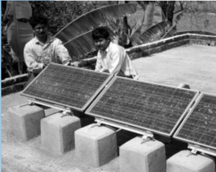
Figure 4.2. Technicians install photovoltaic modules on a village clinic in West Bengal, India.
