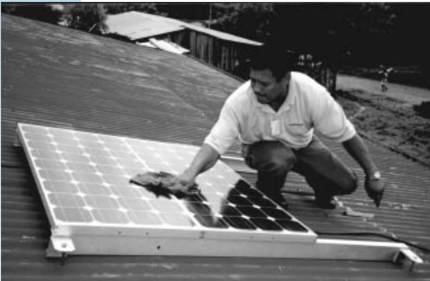
Figure 2.2. A photovoltaic technician cleans two 80-watt panels which power a Sunfrost vaccine refrigerator in the community of Mulukuku, Nicaragua.
