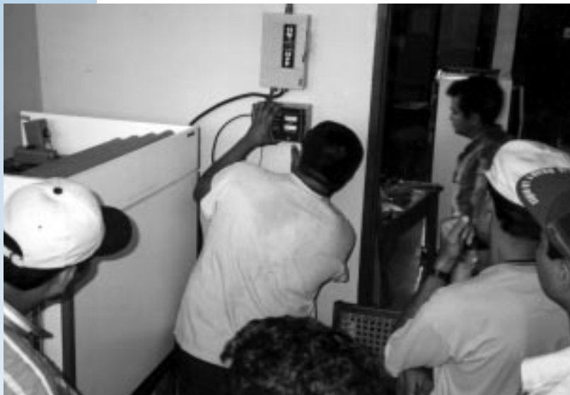
Figure 4.3. A photovoltaic technician's course completes the final installation checklist prior to commissioning a photovoltaic powered refrigerator/freezer at Clinica in the community of Mulukuku, Nicaragua.
