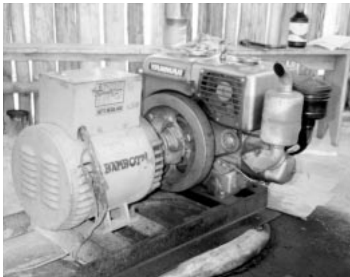
Figure 2.5. A diesel generator is the typical source of power at small rural hospitals. Smaller clinics may rely upon smaller gasoline powered generators for emergency use only.
