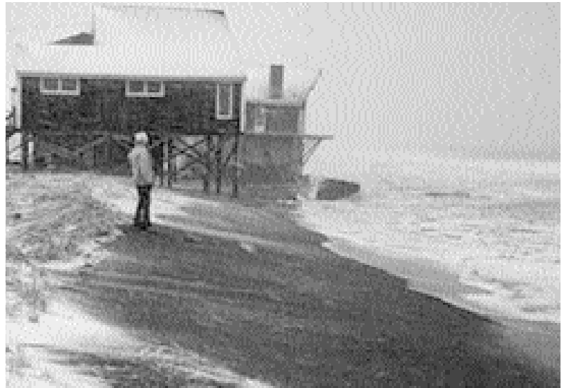
Coastal erosion in Charlestown, Rhode Island.
