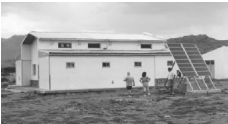
Figure 1.2. PV system, including panels, batteries, and regulator box at a school in Collipilli Abajo, Argentina.
