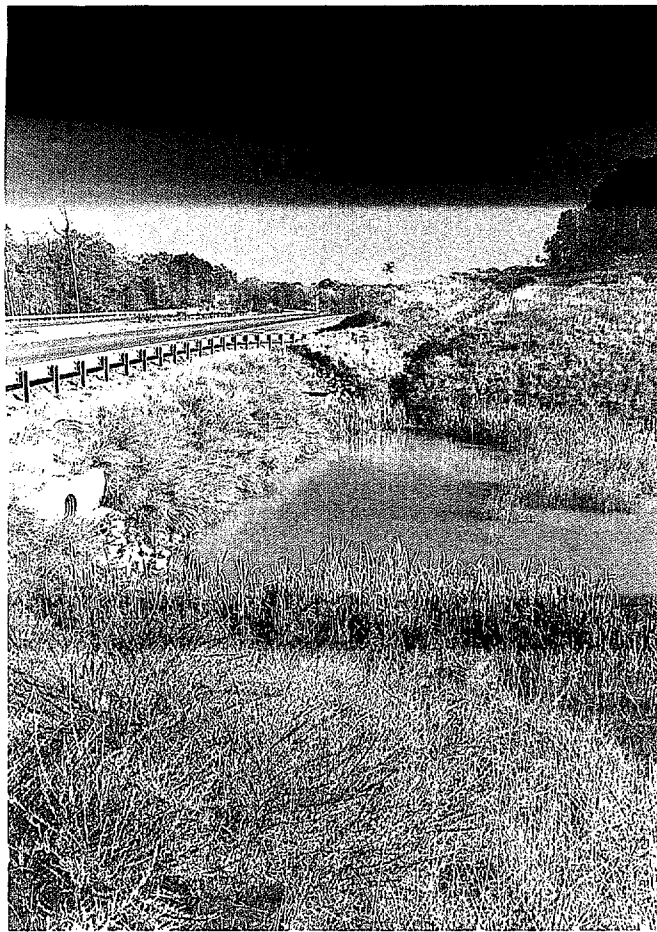
Wetland Replacement Design, Landover, MD
