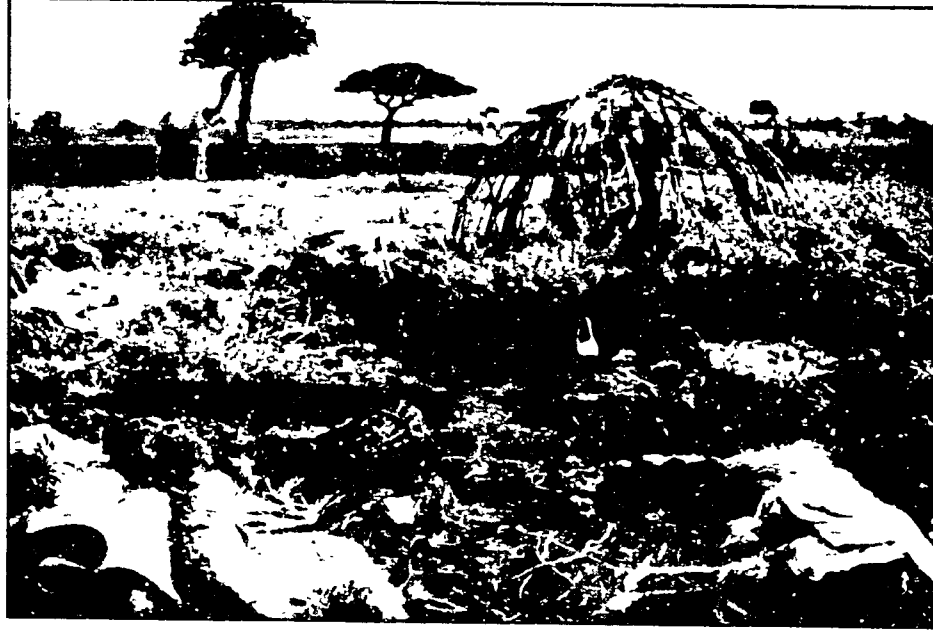
Nomad hut under construction. Material in foreground will cover frame. The entire house was carried by the camel in the background.
