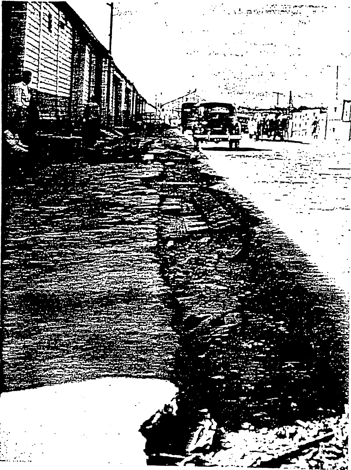
Damage at Suva wharf caused by the 1953 earthquake, which was followed by a tidal wave within 30 seconds.
