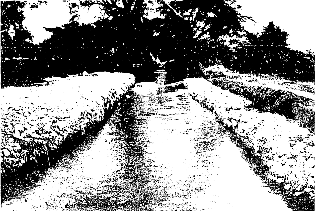
Plate 18 - Part of Rio Cobre showing Groynes to prevent soil erosion.
