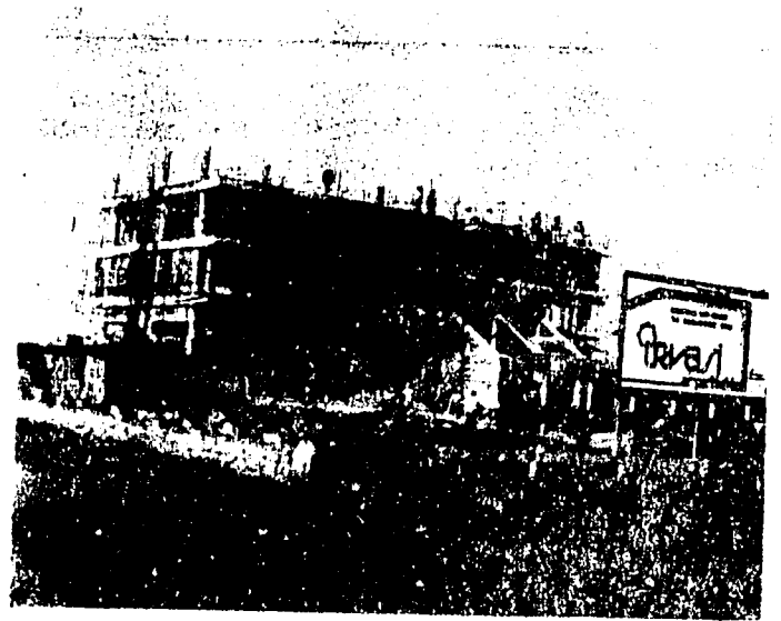
Hotel Urvashi under construction
