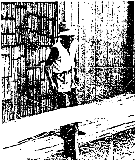
FIGURE 13--Final step in making a bamboo board--removing diaphragm fragments from the newly opened culm. It may be done with a machete, as here, or with an adze or a long-handled, shovellike curved spud.
