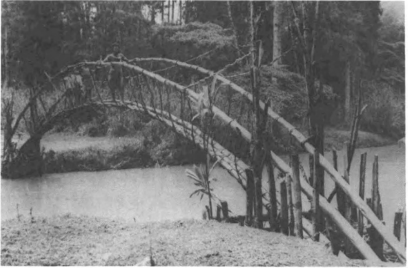
Roundwood. Lagaip River, Papua New Guinea. Flexible young casuarinas joined to form the arch of a bridge. (J. Siegel)
