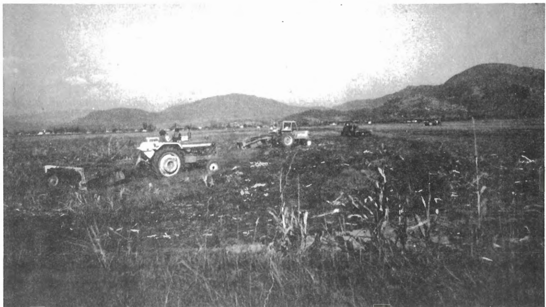
Land levelling by private contractors, with mechanical scrapers, at Dalaman State Farm.
