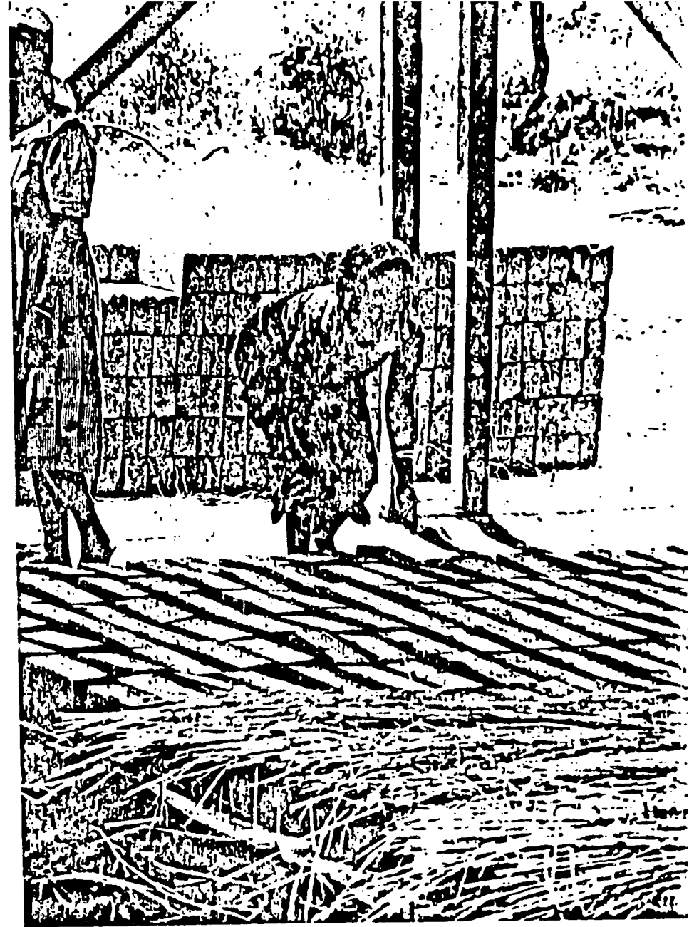
Pressed bricks were allowed to cure for two weeks before going into the walls.
