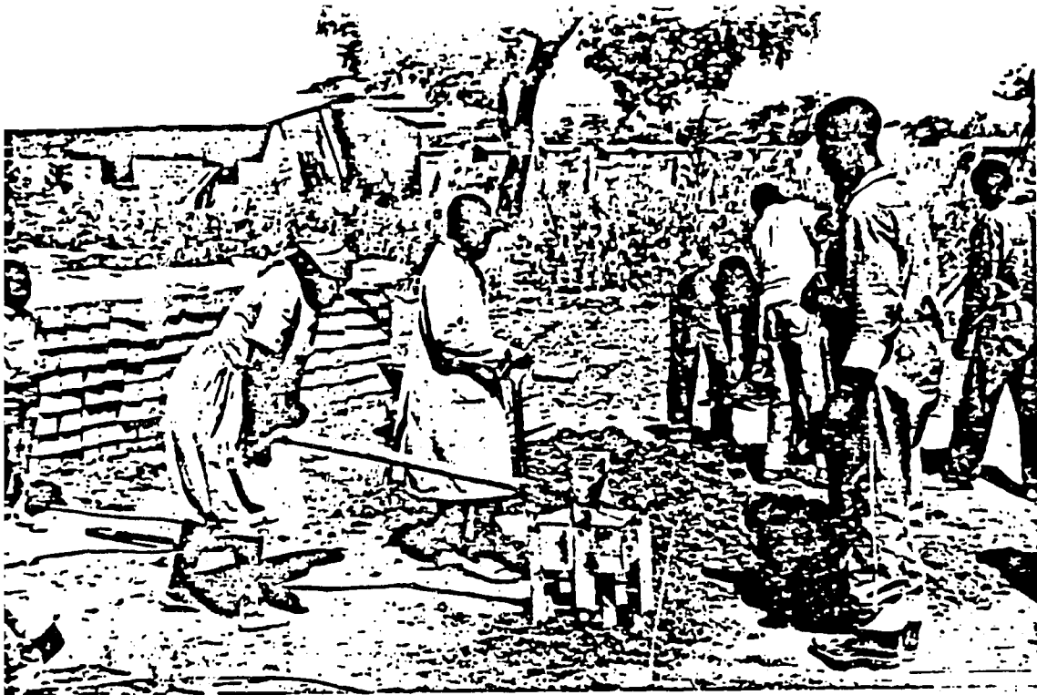
Pressing the earth and cement mixture in the Cinva-Ram which produced the bricks.
