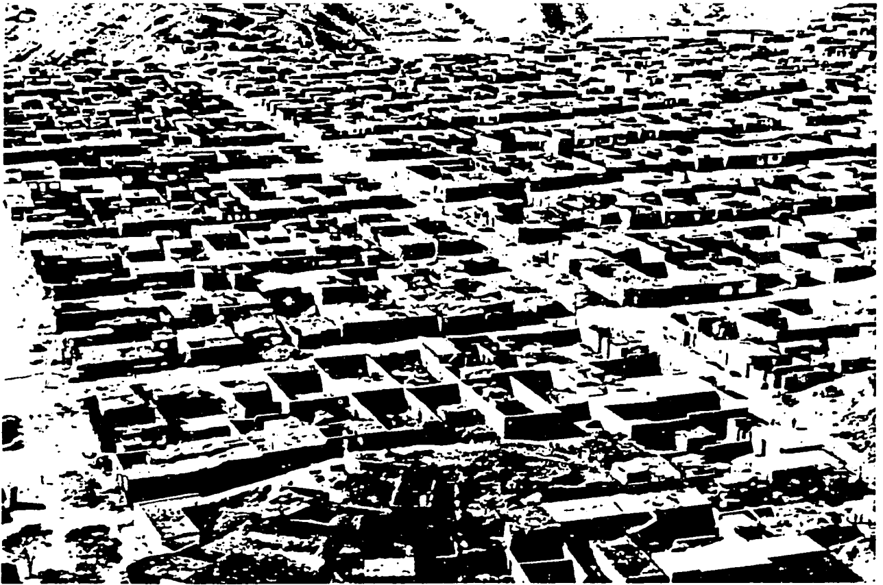
View showing the various stages of house development. Credit: J. C. Turner
