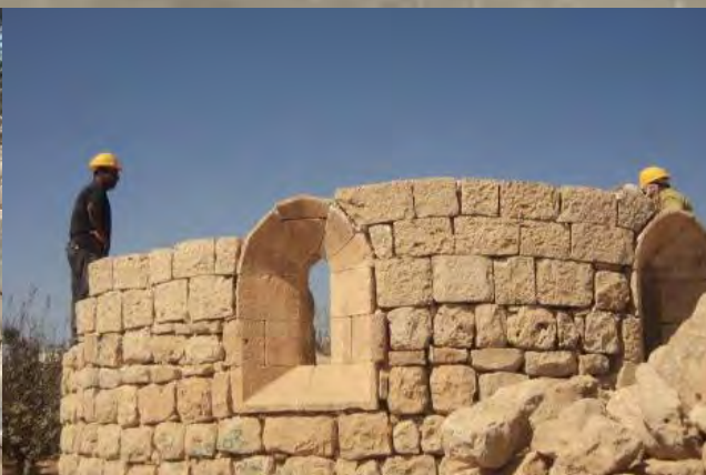
Top: The finished rehabilitation showing the widened road, new sidewalks, relocated tower, and the new retaining wall leading to the tower. Bottom left: The previous road and wall. Bottom right: Workers shifted the stones for the historical tower one by one.
