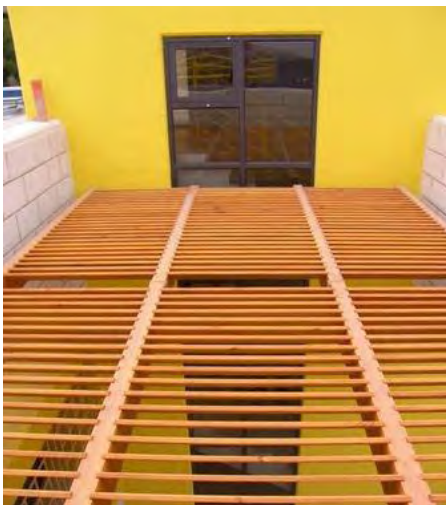
The building orientation and structural window shading reduces heat from the sun.
