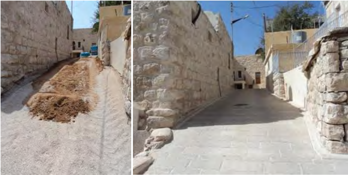
Left: During the renovations in Taybeh and Right: The same path after the renovation was completed.
