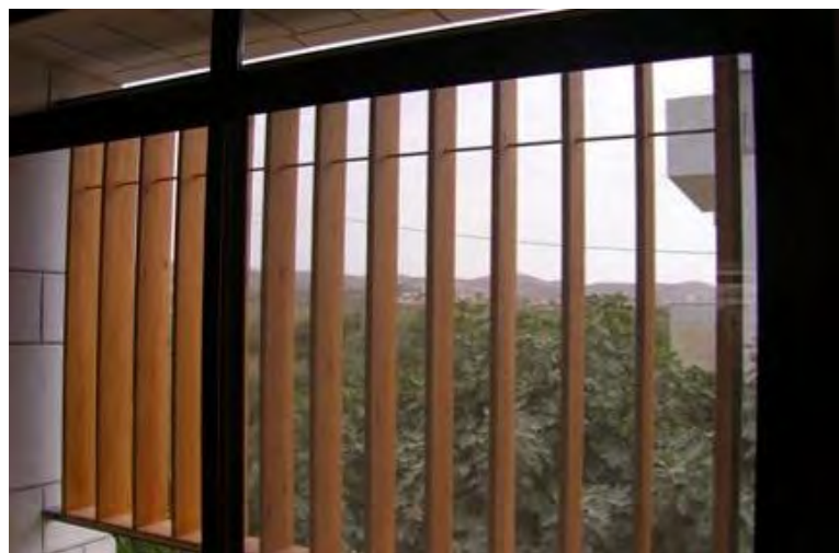
The building orientation and structural window shading reduces heat from the sun.
