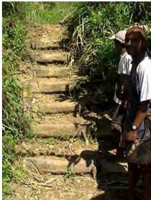
Figure 4: Trail construction at the Andrambovato forest station. The steps for the trails were made out of tree limbs that had fallen in the forest.
