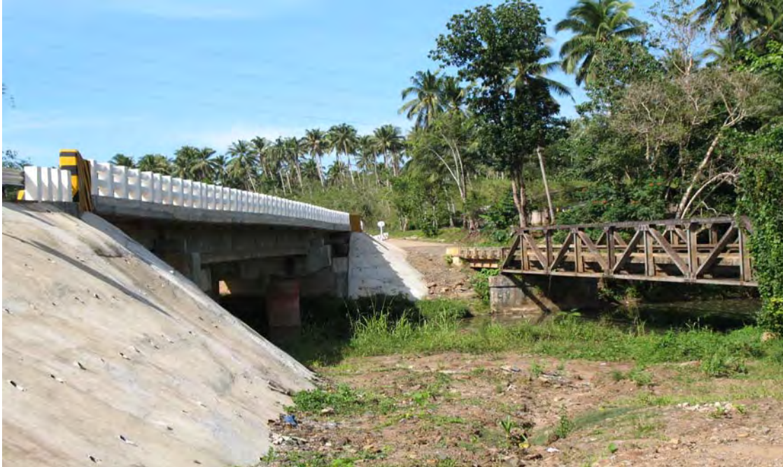
Photograph of a concrete two-lane bridge, a regional infrastructure project, on the Sulu Archipelago island of Basilan. On the right is the old one-lane bridge that was replaced. (Office of Inspector General, February 2008)
