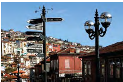
Energy Efficient Street Lighting in Veliko Tarnovo
