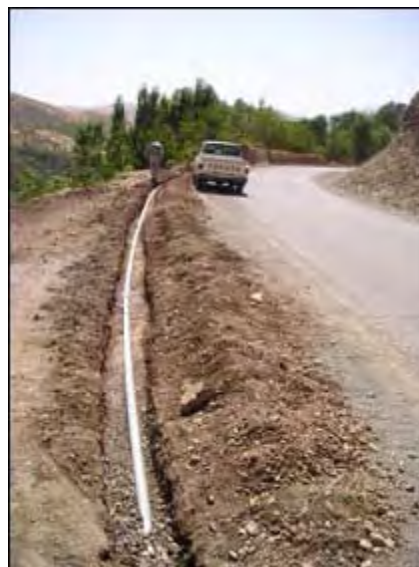
Over three kilometers of pipe laid in 15 days.
