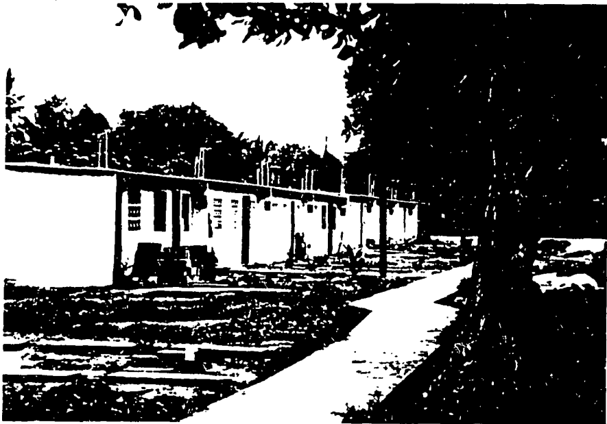
TWO BEDROOM UNITS IN PROTAL SOLD FOR $ 6,500 EACH. THEY CAN BE EXPANDED TO THE REAR
