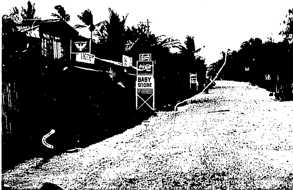
This section of road is typical of the many cases where right-of-way for widening the road was not obtained by DPWH from residents prior to construction. Picture taken at the Kalibo road project.
