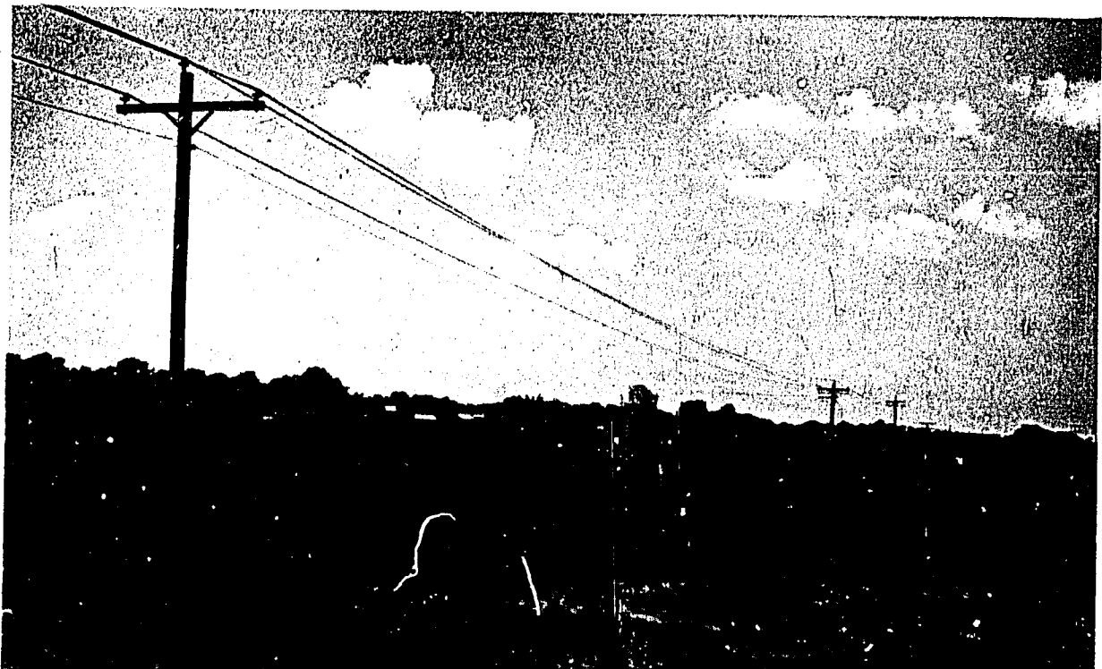
A rural distribution line in operation
