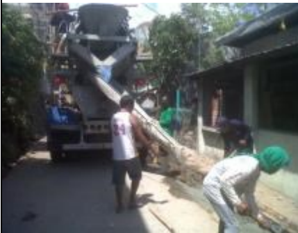
Pipe-laying of distribution lines
