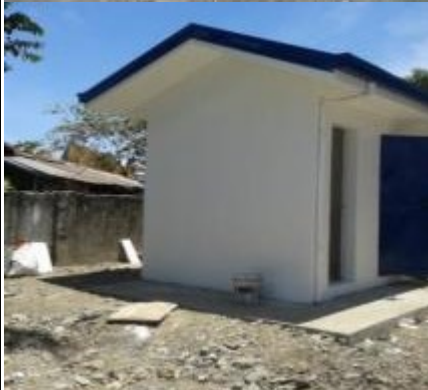
Well head and Pump-house
