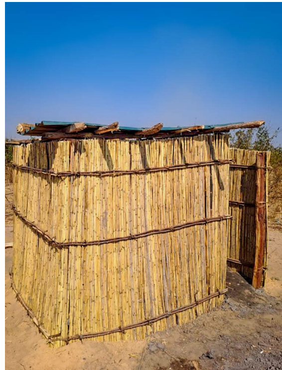
Photo Credit: USAID Expanding WASH: An improved demo Baruto toilet.
