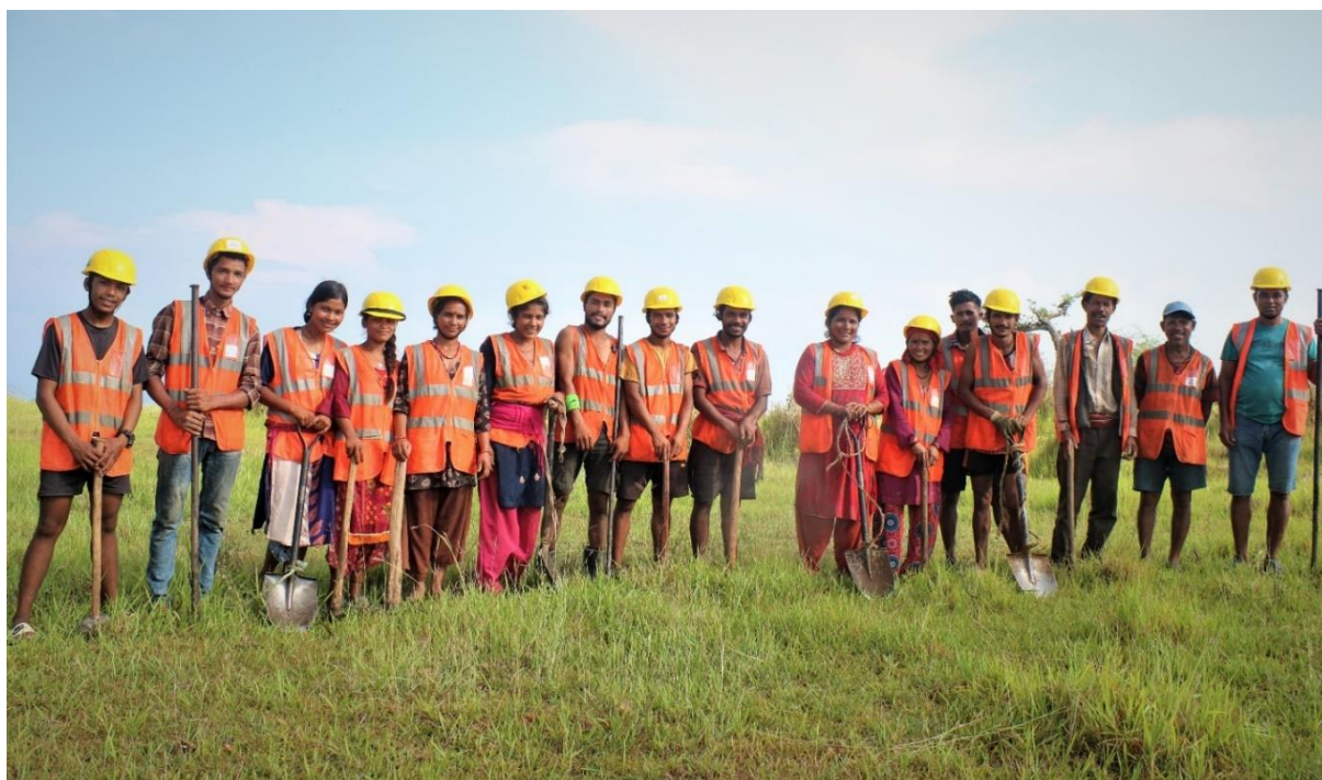
Photo 1: WUSC and community engaged in pipe laying work in Pokharikanda WSS
